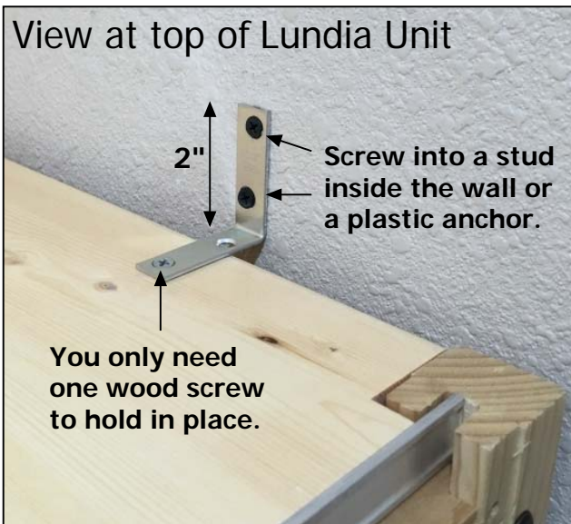
Attach "L" bracket to top shelf and wall as shown.
